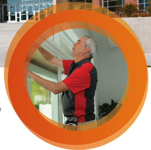
Proper installation of security film is essential to its success. For the best, most effective results the film is first adhered to the inside of the glass then a wet glaze silicone attachment system firmly secures the film and frame together. The combination of the security film and the attachment system provides additional security over a window without an attachment system.
